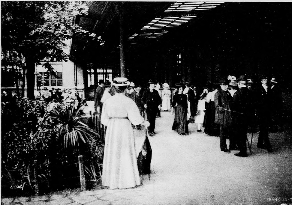
Entrance to Departure Platform, Western Railway Station, Budapest.
