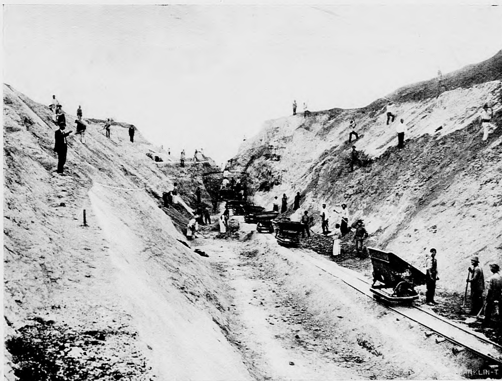
II. Railway Construction near Lake Balaton.
