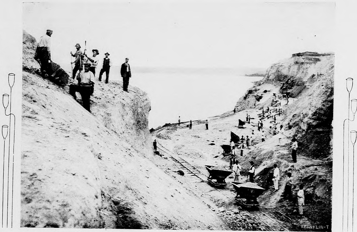
I. Railway Construction near Lake Balaton.
