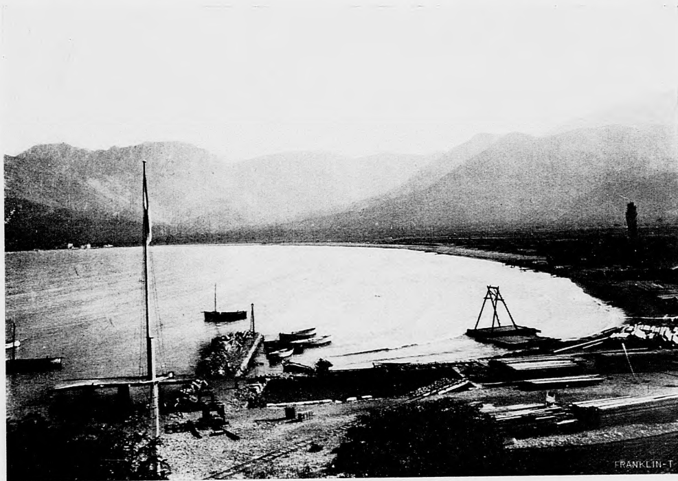
Antivari : Harbour Construction.
