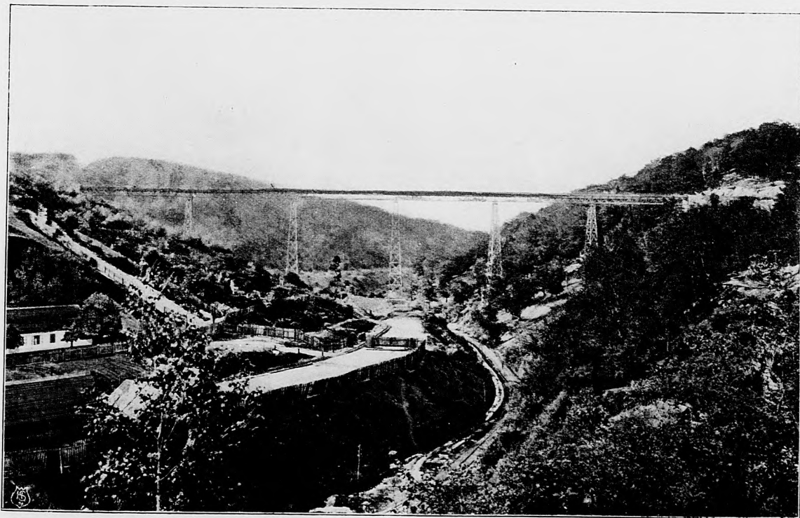
Austro-Hungarian State Railway: Aqueduct at Szekulo.
