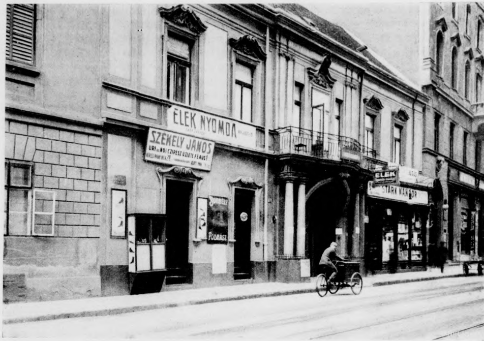
Vanishing Budapest: Old Houses now being Demolished.
