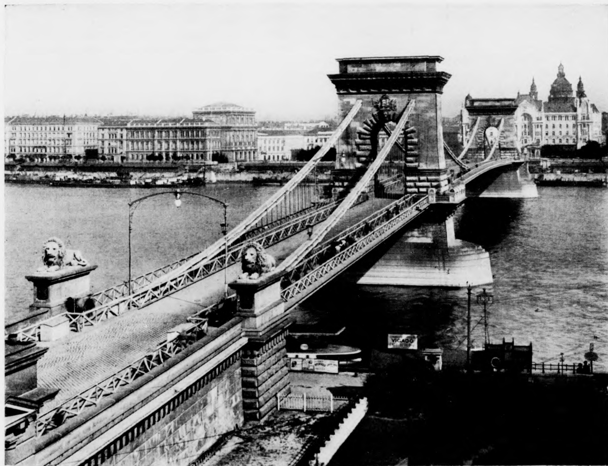
Suspension Bridge, Budapest.
