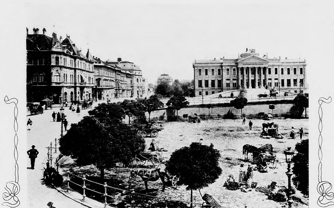
Tisza Embankment, Szeged.
