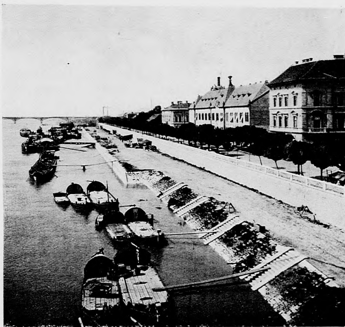
Tisza Embankment, Szeged.
