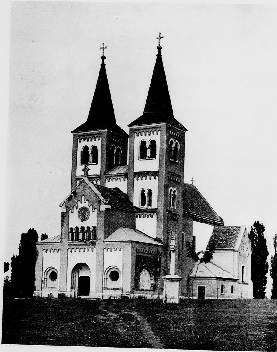
The Church at Bény. Restored in the XIIIth Century.
