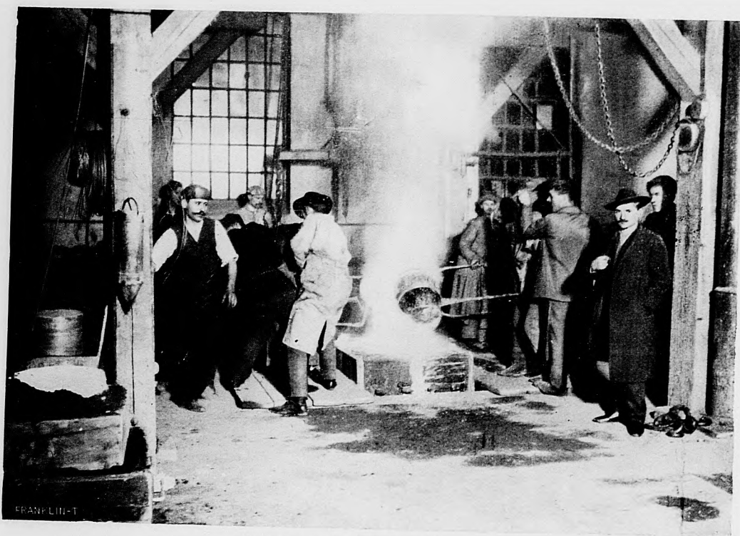
Pouring out the bronze in the mould.
